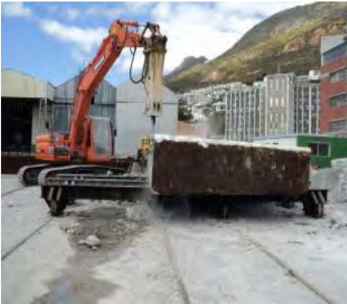
Demolition of TRANSNET Iron Ore Sampling Plant 30m Steel Structure 2013
