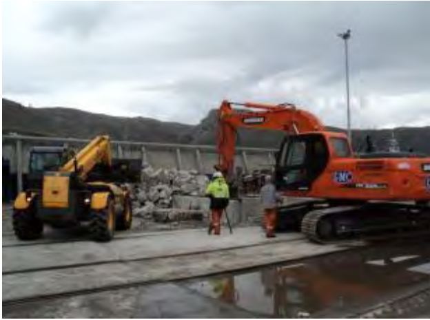
Demolition of Sierra Wall Cutting the concrete wall into sections and floating away to be demolished 2012 SIMONSTOWN
