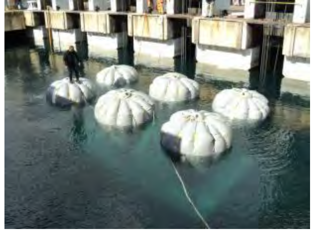
Demolition of Sierra Wall Cutting the concrete wall into sections and floating away to be demolished 2012 SIMONSTOWN
