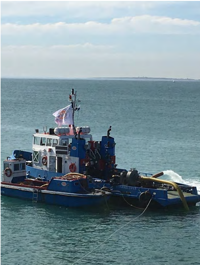
Dive Support for construction of trench
