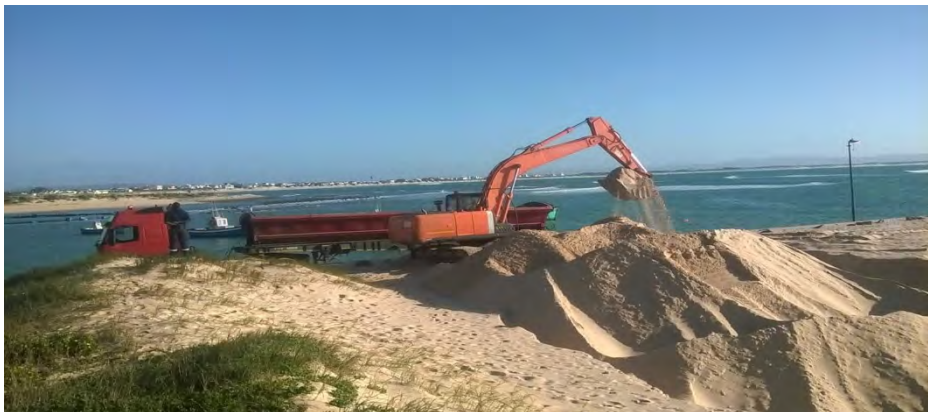
Removal of dredged material in Stillbaai using a 30 tonne excavator.
