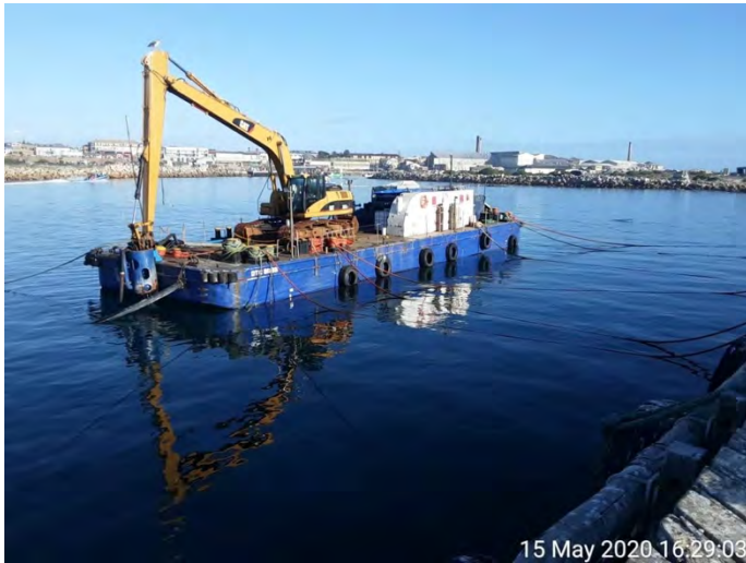
30 Tonne long reach excavator on Barge Franco with DOP pump Power Pack Dredging in lamberts Bay.
